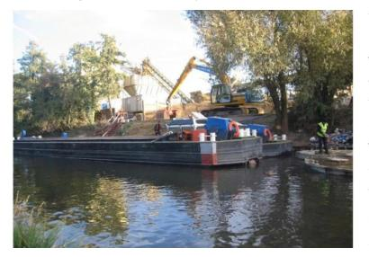
the freight carrying capacity. About 70 tonnes - over three lorry loads – were taken in each barge. Extensive dredging had been carried out so that the barges could load to over 4ft 3" draft. The barge holds were fitted with an inner "skin" with sloping sides, allowing the grab to unload more effectively the last few tonnes.
