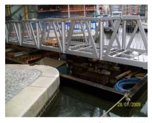
In another example a hydraulically operated lift bridge that had been installed in Paddington before the recent developments took place needed to be removed for servicing. The only access to this bridge was from the canal. Using a plant pontoon, a lifting turntable allowed the bridge to be lifted up off its fixings and to be rotated round 90 degrees and lowered into the pontoon. It was then moved along the canal to an access point for onward transport by road.
