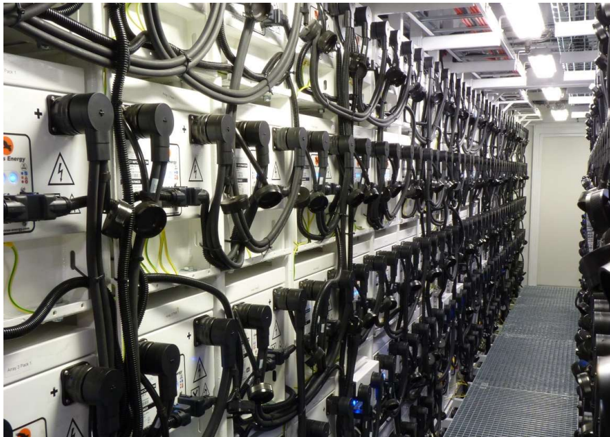
Typical Battery Installation
