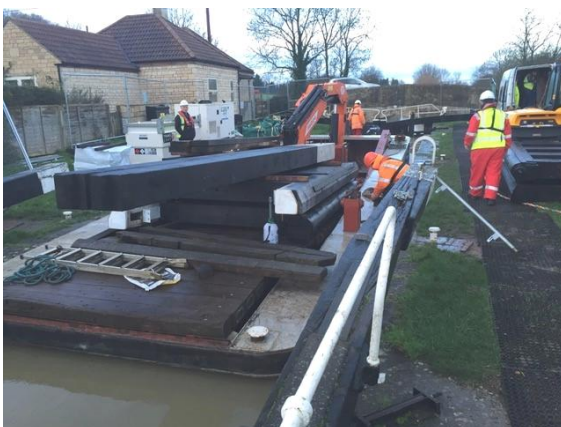
Gates arriving by barge at Seend Lock, Kennet and Avon Canal, January 2016 (C&RT)
