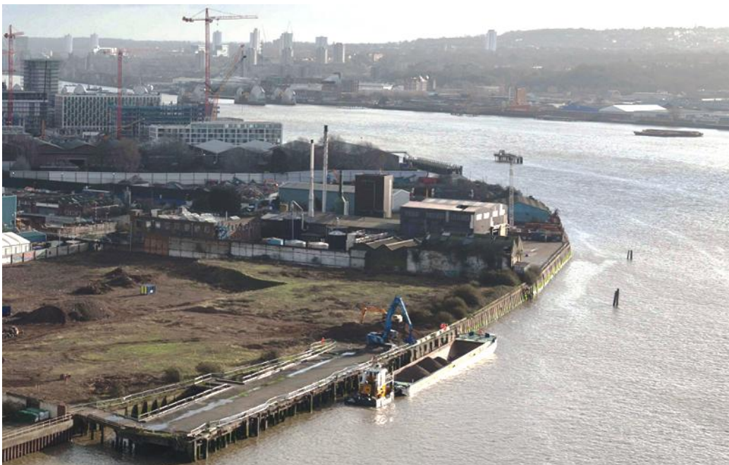
Peruvian Wharf showing a barge and preparation work underway for future use. The Thames Barrier can be seen in the distance. (PLA)
