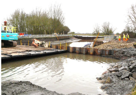
Aire and Calder breach near East Cowick with piling across the navigation so that the cause could be assessed (Stuart McKenzie/Canal and River Trust)
